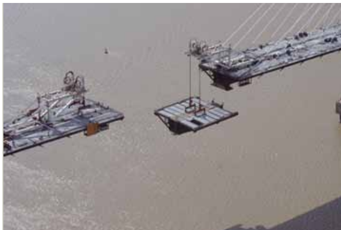
The team used a hydraulic lifting and skidding system
